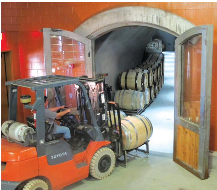
The cave is 15 feet wide with an eleven-foot ceiling and has two potential entertainment areas (19 feet wide with 14-foot ceiling). Floor has a 2% slope for drainage. A sprayed-on impervious layer sandwiched between seven- and nine-inch thick shotcrete layers acts as a water seepage system for the walls and ceiling. The cave was constructed through wet-squeezing clay by Nordby Wine Caves (Santa Rosa, CA). Monitoring systems were employed during excavation to monitor movement due to expansive soils. There are two external and one internal (shown) access portals.
