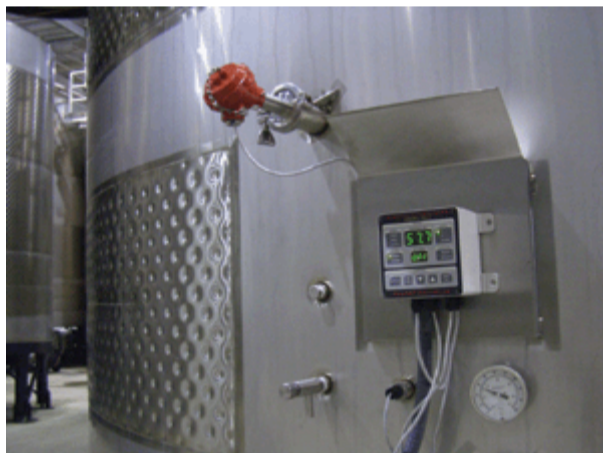
TankNet controller reading a brix probe at Monterey Wine Company.
